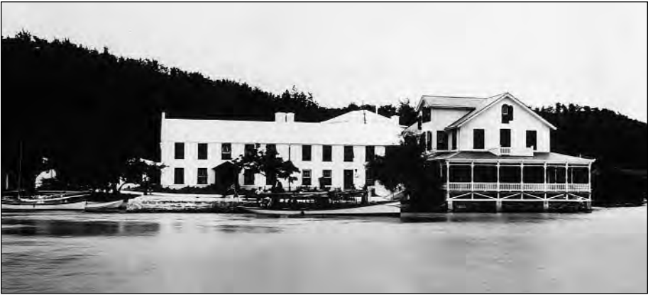
The Hotel Frascati in Flatts, photographed here in the early 1900s, was BBSR's first home
